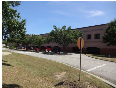
Robins AFB, GA ($8.0M Const. Cost) 147,500 SF. Security Forces Building
